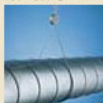
Wrap cable around Spiral duct
